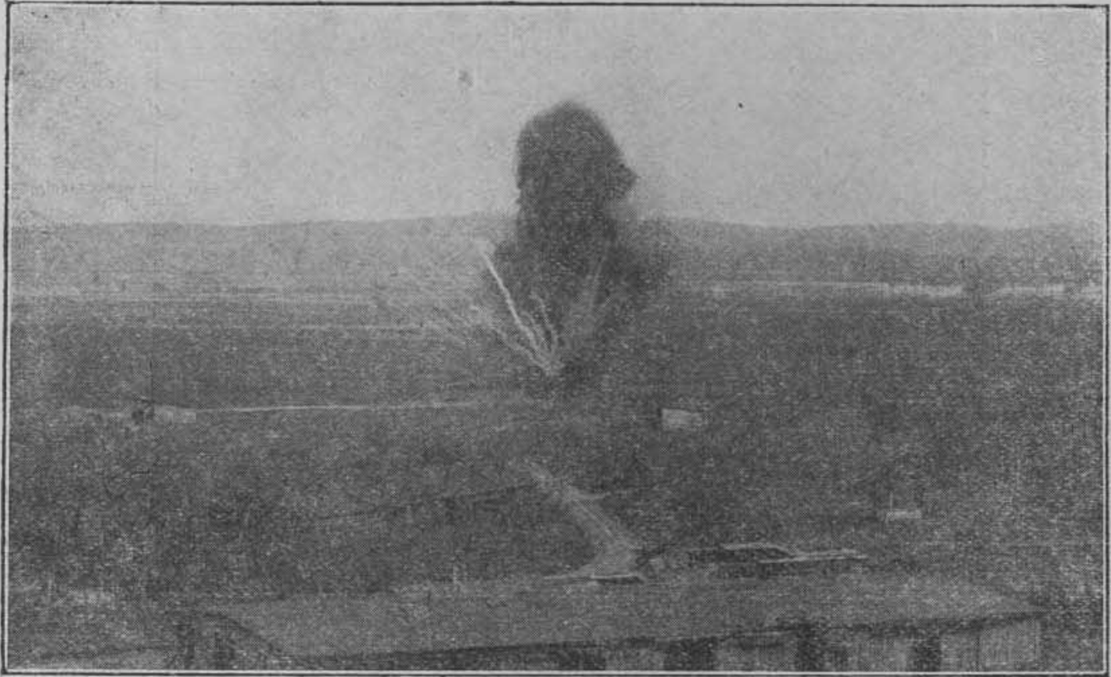
One of the most interesting post-Armistice accomplishments of the Ordnance Corps was the cleaning up of the army areas and the demolition of ammunition. The shells were carefully piled in shell holes or any depression in the ground and dynamite or some of the more sensitive shells or bombs placed on top of the pile as a detonating charge. The fuse led to a fulminate detonator in this charge.
